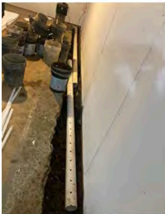
Inside footer tile for under slab drainage.
