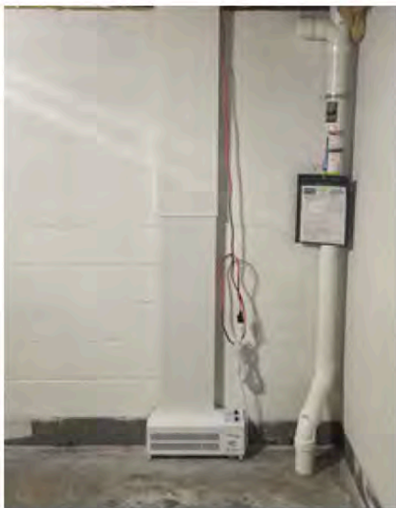
EZ Breathe Ventilation System and Radon Mitigation System.
