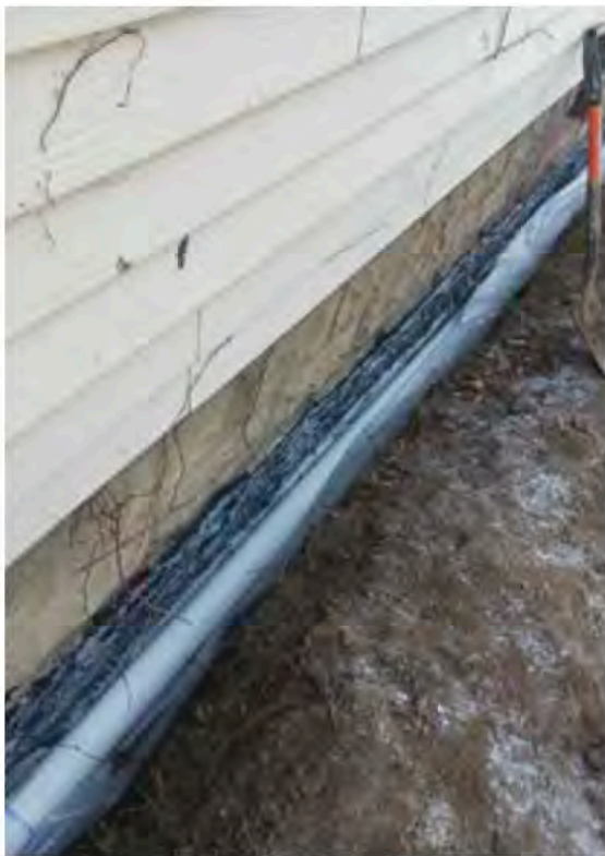
Complete installation of subsoil drainage system along exterior foundation.
