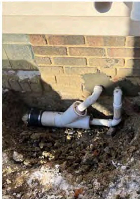
Output from internal pump discharge lines to exterior storm line.
